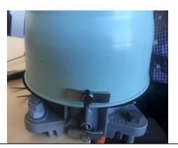
**Note:** An extra entry port is provided in the Moisture Barrier for the 6mm<sup>2</sup> Earth and Service Cable. These need to be disconnected and passed through the entry port in the barrier.
